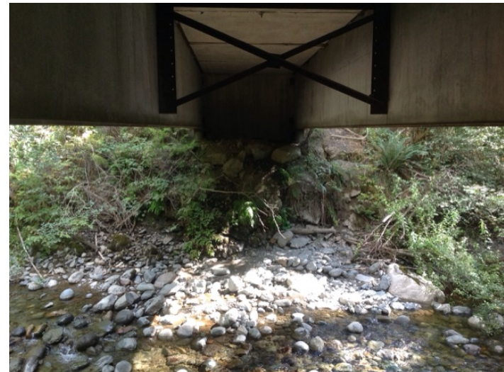
Left Bank Abutment when facing downstream
