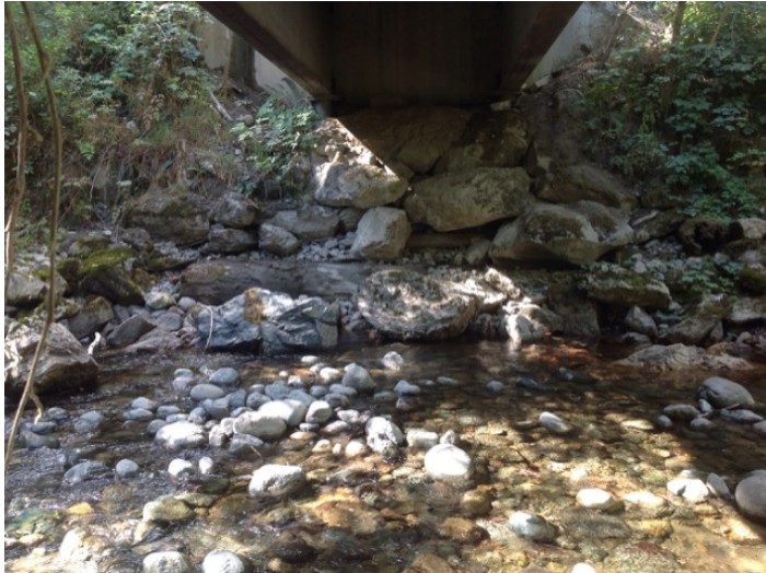
Right Bank Abutment when facing downstream
